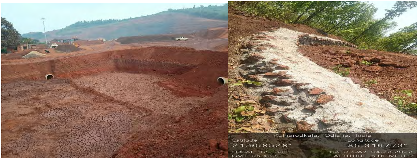
Retaining wall/Garland drain/Settling Pond
